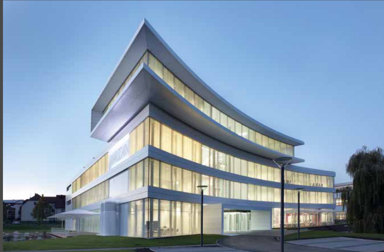
Marc Cain Headquarters, Germany | Architects: Hank und Hirth, Germany | Material: ALUCOBOND® plus White 16
